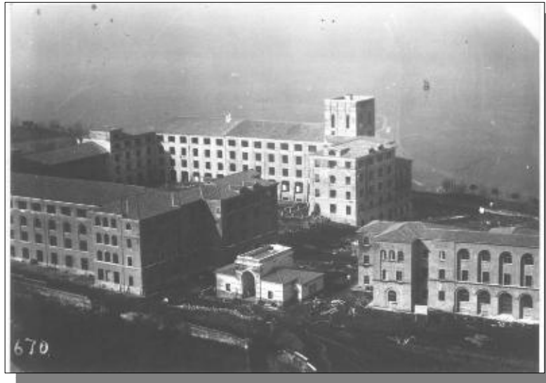
Fig. 2 PIAVE Barracks of Orvieto. Photo of Archive
