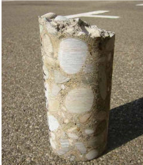
Fig. 10 Concrete carrots from B3 columns
